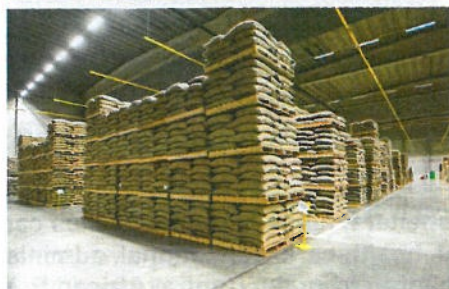
Temperature and moisture levels at Seabridge are continuously monitored and the air is filtered
